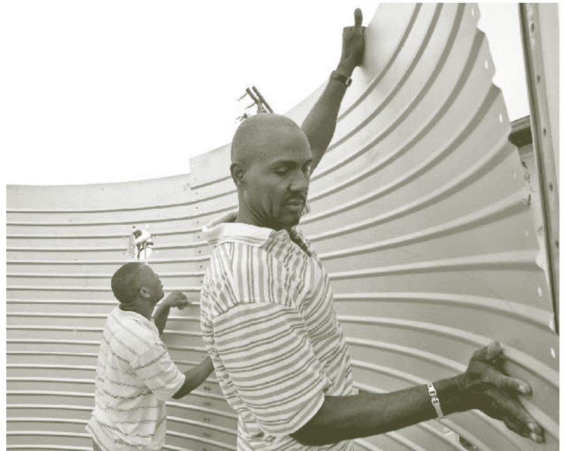
Haitian workers add the second series of panels to a 20,000 liter water tank in the Acra camp in Port-au-Prince. After the sheets of zinc are bolted to vertical ribs around the structure, a plastic lining makes the structure waterproof.
