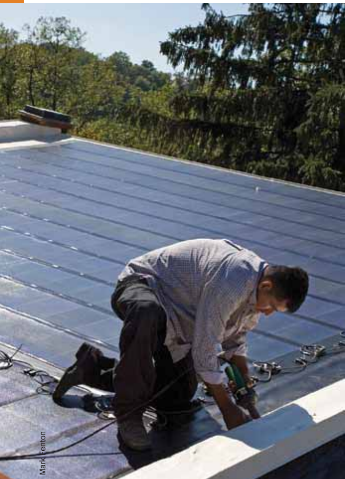
A worker installs a solar roof on a home in the District of Columbia.
