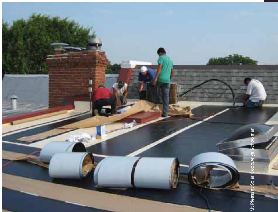
Roofers install solar panels on a home in the District of Columbia.
